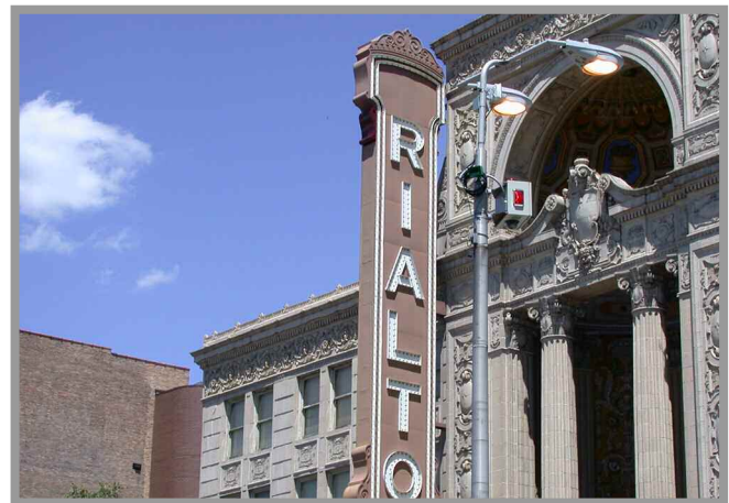
Temporary installation of ARVIS with IK-DP30A camera at Rialto Theater (Joliet, Illinois)
